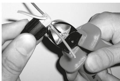
4. Protruding cables are flush, i.e. cut off **to size**. Use a wire cutters for example to do so.
