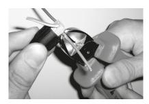
Protruding cables are flush, i.e. cut off to size. Use a wire cutters for example to do so.
